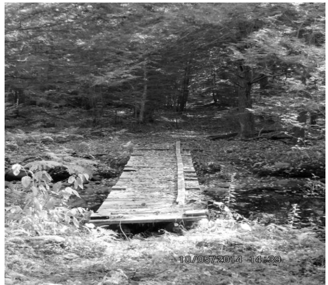
New Boston Road Conservation Area Bridge
